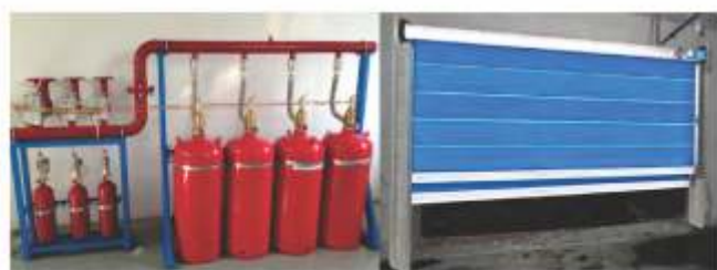
NETWORK TYPE FM200 FIRE SUPPRESSION SYSTEM (HFC 227a)
